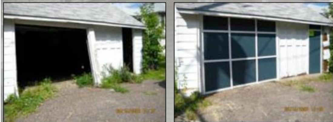
These are examples of before and after photographs of structures boarded in Artistic Board-up manner. The after photographs show that the material used to secure the opening was painted in a manner as to represent the original covering. Artistic Board-up presents a uniform presentation. In many cases the Artistic Board-up looks better than the original window or door that it is replacing.
